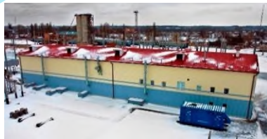
2006-07 Installation and adjustment of traction substation Poltava
