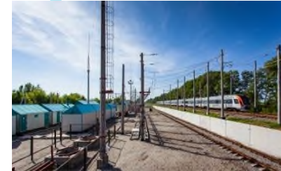
2011-12 General contractor of construction of traction substation of Grebenka - Poltava-Krasnograd - Lozovaya site
