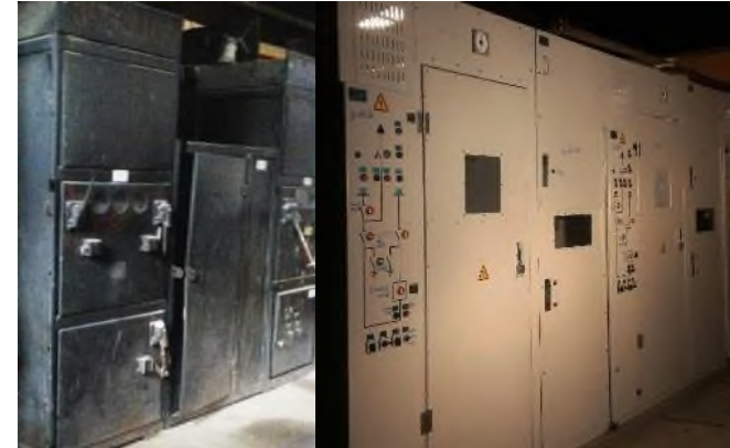
Rehabilitation of SG-3,3 kV RS Khresili, Georgian Railway
