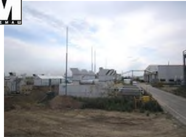
Equipment for power supply for machine-building factory in Atyrau city, Kazakhstan
